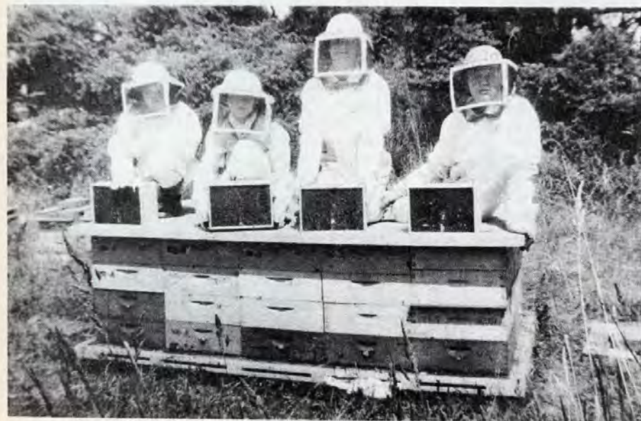
Roy, Glen, Bill and David behind beehive condominium...showing supers 4-deep...and packaged bees on top. Note the 3/4 inch plywood roof and floor both have edges reinforced with 3 more layers of the same plywood, for extra resistance against bears.
