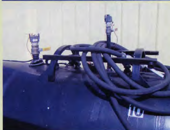
Compressed air is fed into the feeder tank, and it pushes out syrup.
