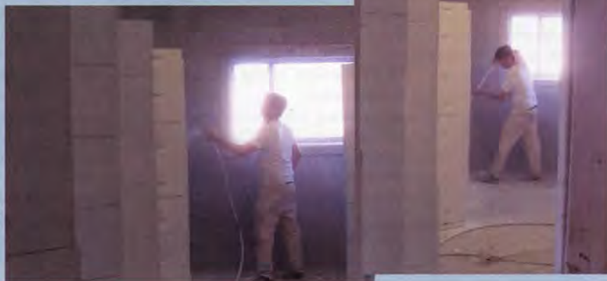
. . . and finally, two coats of latex are applied.
