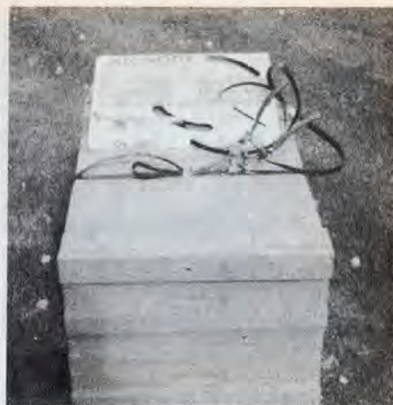
Signode plastic strapping, cutting and tensioning pliers, model DLT and Adams tensioner (on carton).
