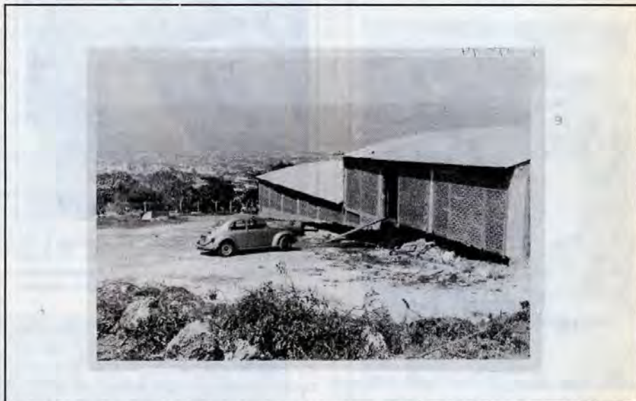
PHOTO 1. Tirado's new extracting plant overlooks Tuxtla in the Grijalva Valley below. The Chiapas Highlands rise beyond. The plant is in two levels, with extraction taking place on the upper, and loading of barrels of honey occurring below.
