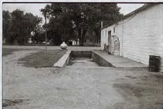
The single loading bay at the Bruce plant. Full supers are unloaded and moved into the hot room, right inside the door. Empties are moved out the same door.
