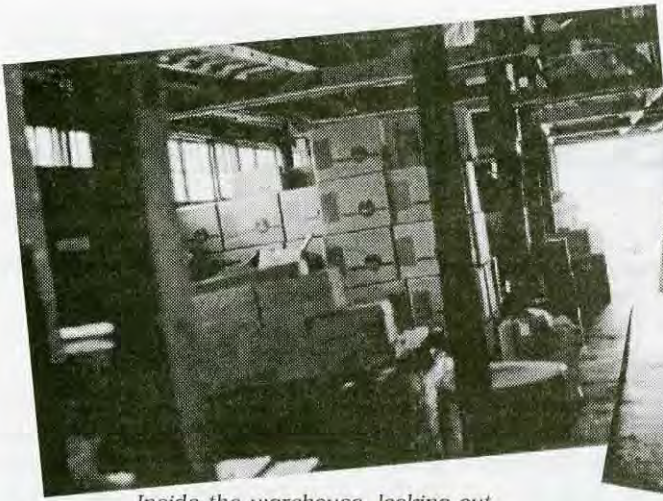
Inside the warehouse, looking out.
