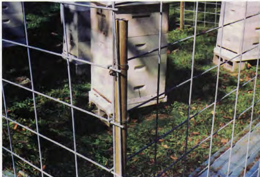
Fiberglass posts with nut and bolt fence panel supports.
