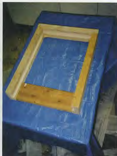
Bottom board before installing screening and leveling board. Photo 4.
