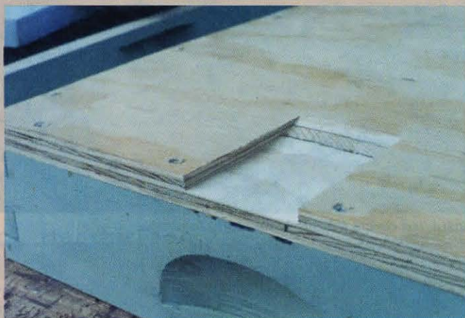
Dado cut for the entrance and ventilation
