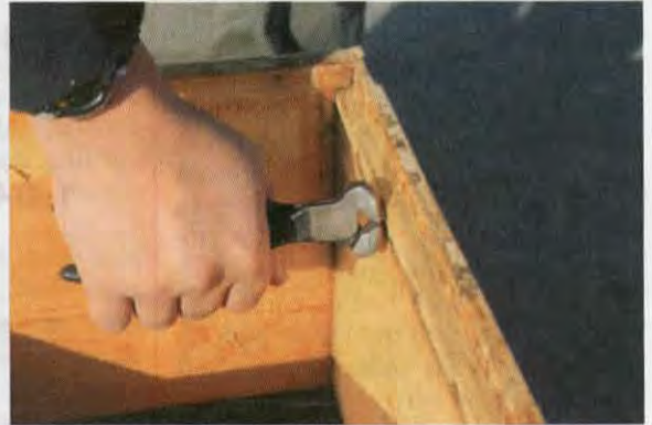
Remove any remaining nails.
