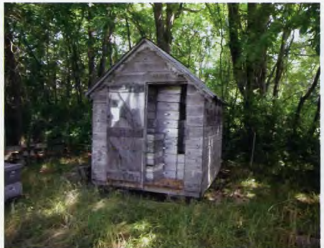
A typical storage shed that comes apart. Some are made of wood, others tin, but each has a floor, front, back, two sides and a two-part roof, and all the parts fit on the company truck.
