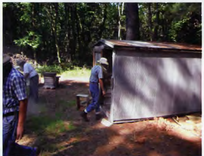
Another shed, this one made from corrugated tin sheets and lumber framing.
