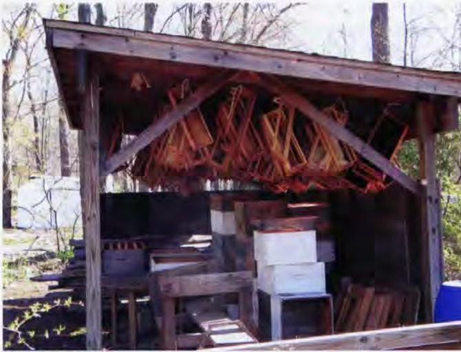
*This open structure found on the grounds of the Pfeiffer Center for Bio-dynamic agriculture in New York state makes use of sunlight and ventilation to allow empty unused frames of comb to be stored year-round without damage from wax moths or mice.*
