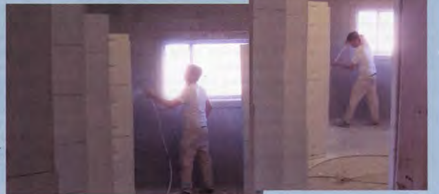
. . . and finally, two coats of latex are applied.
