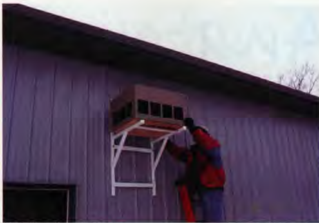
Installing the condenser.
