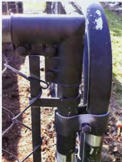
Detail showing the corner bracket, stretching bar, and stretching clamp.
