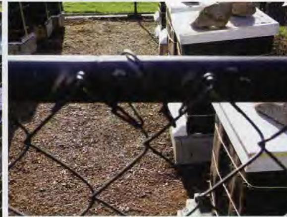
*Clips to hold chain link top and bottom.*
