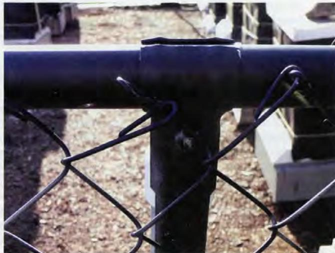
Tee bracket for vertical pipe on panel.
