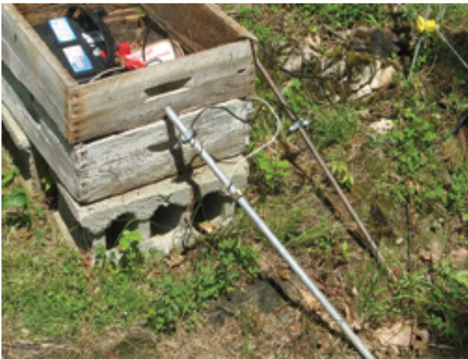
*This electric fence was installed around an apiary located on a rocky ledge which prevented the grounding rods from being buried in the ground to the appropriate depth. Note that the rods are too close together and one of them is made of copper and is likely to fail as the metal corrodes over time.”*
