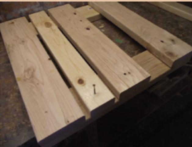
**Step 5:** Now fill in the top by screwing two of part #2 into the gaps between the middle and edges formed by parts #1.
