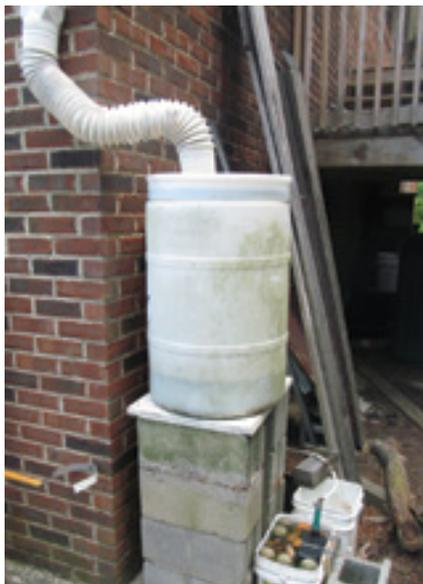
*A clever watering device using captured rain runoff.*
