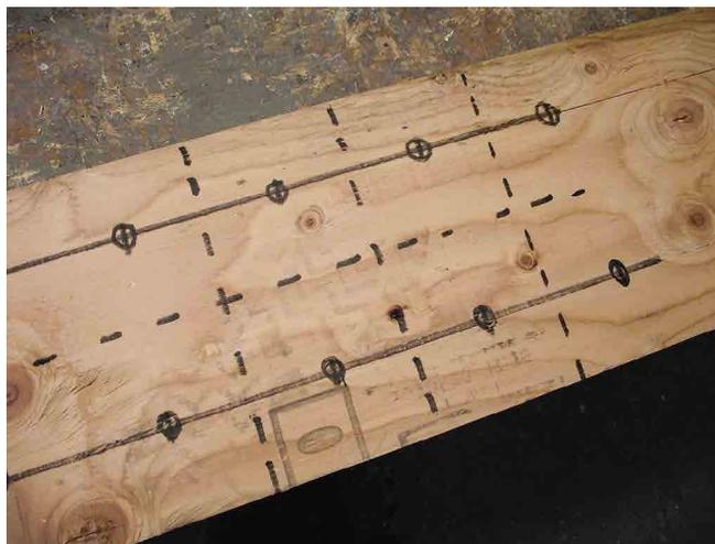
**Step 2:** Now mark the cross line for the centers by starting 2" in from one end and then marking every 4". Do this on both of the center lines marked in step #1. The picture shows the drill marking as circles and the cutting lines as dashes. You do not need to mark the cutting lines. They are there for illustration purposes only.
